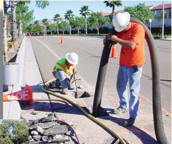
Above: Underground Solutions, Inc. uses air excavation and vacuum rigs to find underground utilities. *See page 27*
